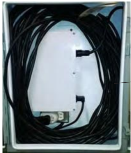
Coil Excess Cable Inside Electrical Box
