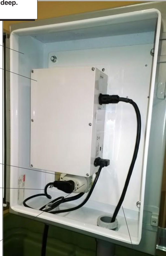
Integrated Power Supply Unit (IPSU)
